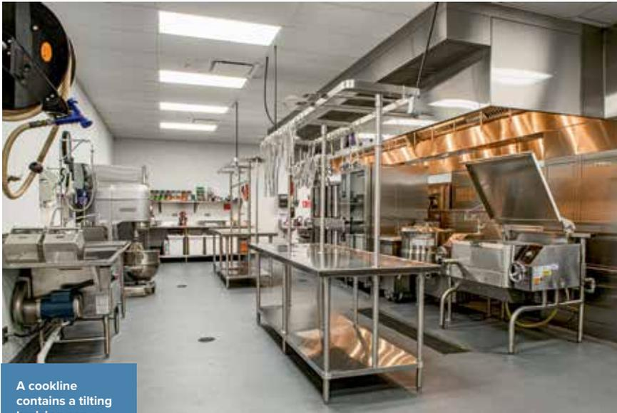
A cookline contains a tilting braising pan, a steam-jacketed kettle, a fryer, a combi oven and two double-stacked convection ovens. The 80-quart planetary mixer and vegetable wash sink sit to the left of the prep tables.
